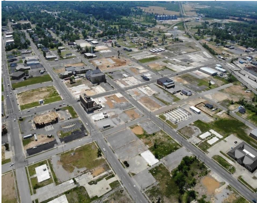
Aerial photo of Mayfield following debris removal.
