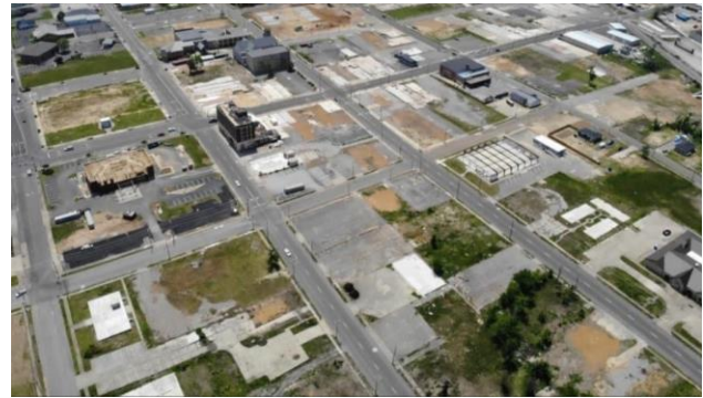
Aerial photo of Mayfield following debris removal.
